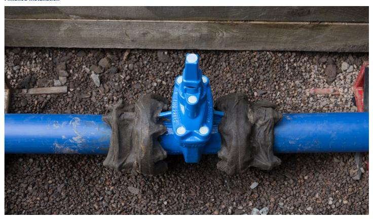
FLANGED GATE VALVE WITH TENSILE RESISTANT FLANGE ADAPTERS, SDR11 PIPE LINERS MANUALLY FIXED ONTO A DN100 INDUSTRY STANDARD PE WATER PIPE, AND WRAPPED WITH DENSO TAPE.
