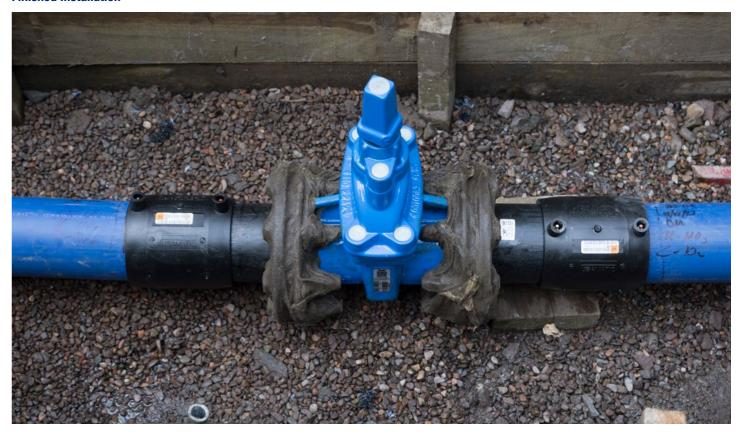
A FLANGED GATE VALVE WITH PE STUB FLANGES AND ELECTROFUSION COUPLINGS FUSED ONTO A DN100 INDUSTRY STANDARD PE WATER PIPE, AND WRAPPED WITH DENSO TAPE.
